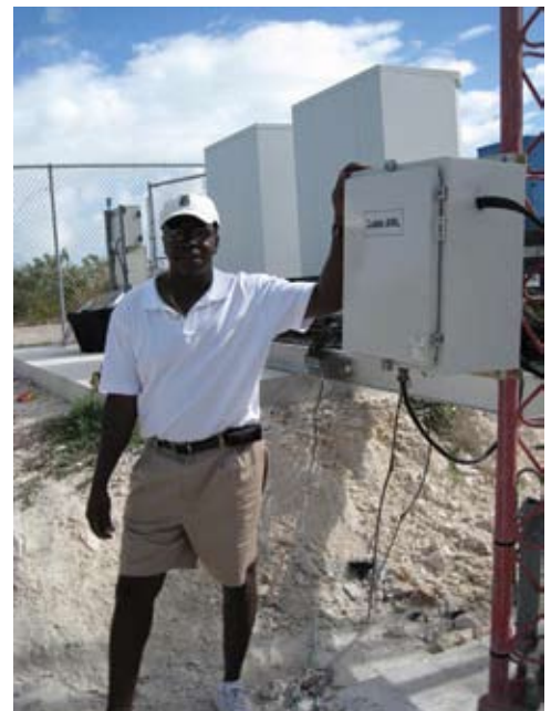
Herbie Ingham following installation of an outdoor Repeater.
