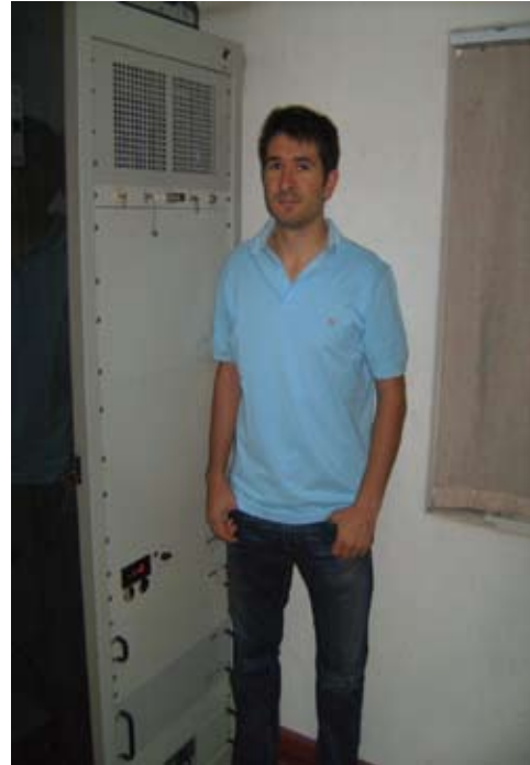
Humberto Barros following installation of the 500 Watt Base Station Transceiver
