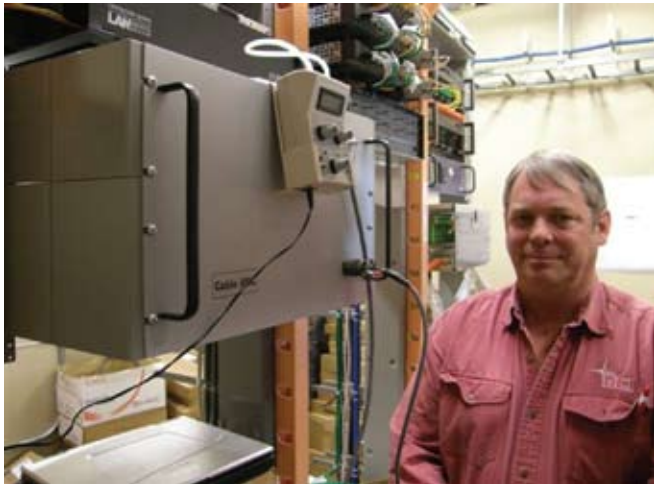
Rick Bates following installation of the Cable AML broadband transmitter
