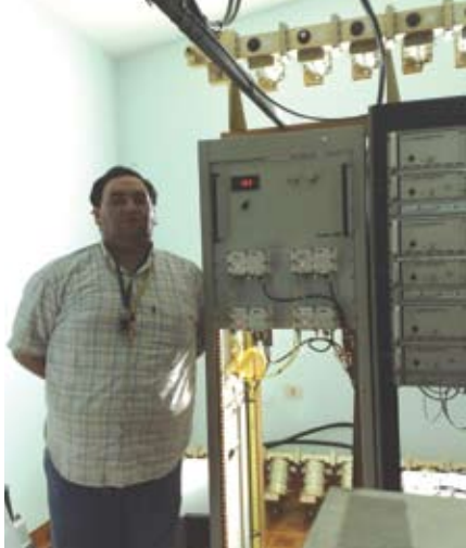
Carlos Esteche following installation of Base Station equipment (the CMTS is 25 Kms away, connected by fiber)
