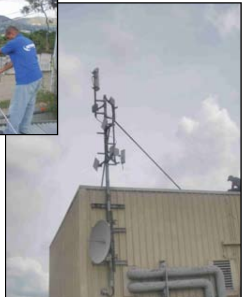
RIGHT: Repeater Site Installation
