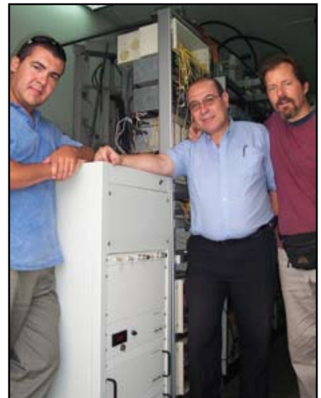
Ing. Javier Montagne, Claudio Bozzo and Fernando Heredia following installation of the new broadband transmitter.
