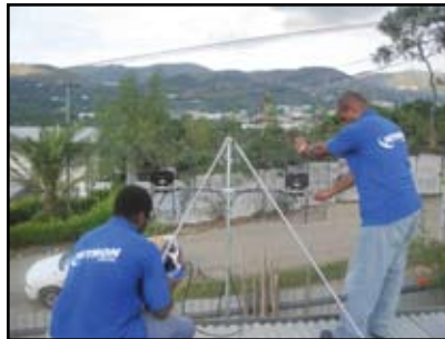
ABOVE: Hitron technicians install antenna at a customer site.
