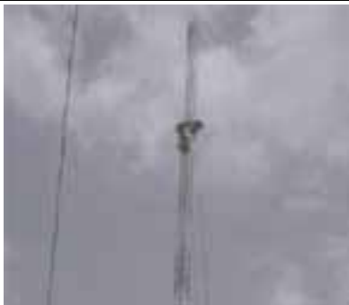
The top of the MMDS transmission tower at the Nanasat headquarters.
