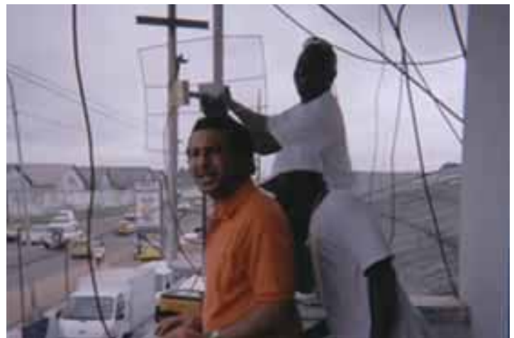
Salleh Hawaidi supervises an MMDS subscriber installation
