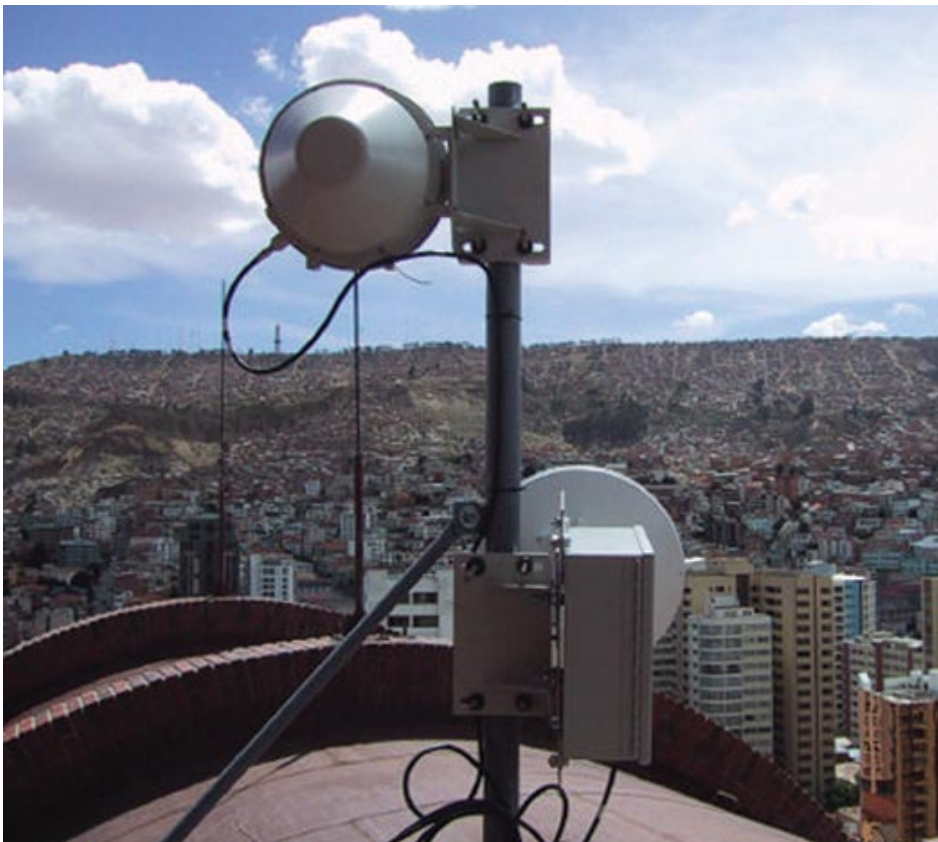
Typical subscriber CPE Integrated Antenna/RF Transceiver installation for 28 GHz LMDS System
