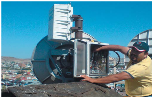
Arturo Perez from Grupo Caliente adjusting one of the new AML receivers.
