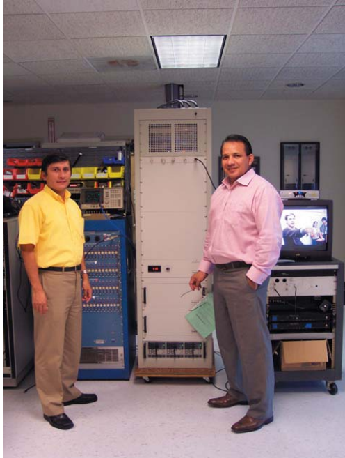
Ing. William Arcentales and Ing. Angel Vacacela during system acceptance testing at Cable AML.
