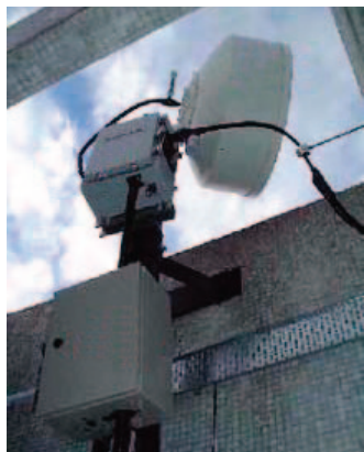
18 GHz Repeater with Input Antenna.
