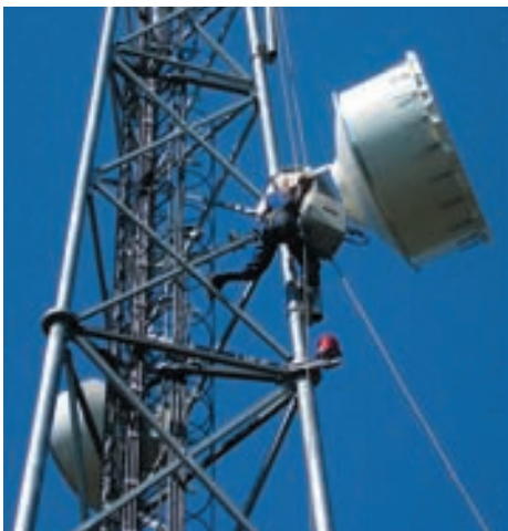
TTT personnel install one of the STL antennas.
