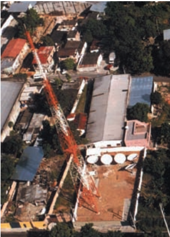
Aerial view of ACOM's headend and transmitter tower in Manaus, Brazil.
