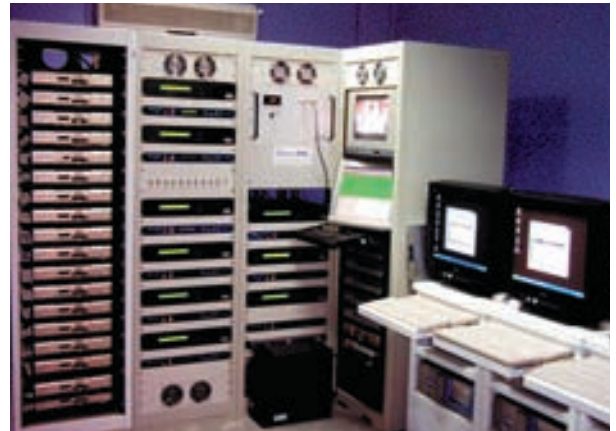
Cable AML's integrated digital headend and broadband MMDS transmitter.
