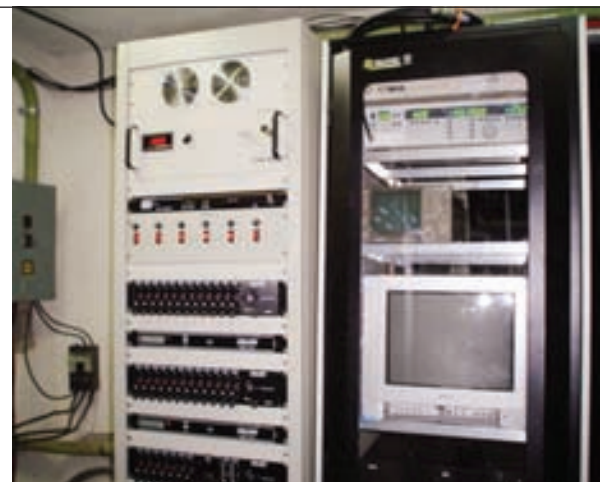
Broadband MMDS System installed at MVS, Mexico
