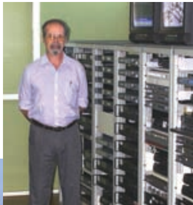
Rafael Horodezki installed the Cable AML system in 1992.
