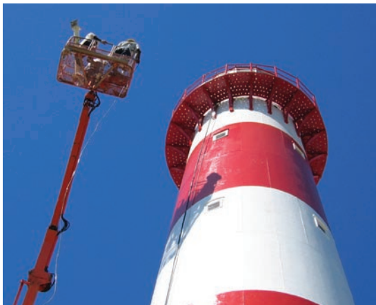
Installation underway at lighthouse repeater site
