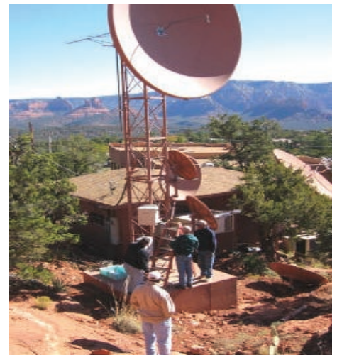
Installing the Return Path Receiver at the Sedona Headend site
