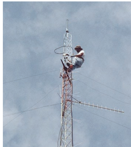
MVS technician installs MMDS antenna in Ensenada.
