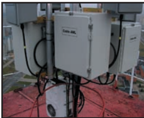
Outdoor wireless DOCSIS upstream receivers installed in Lithuania.
