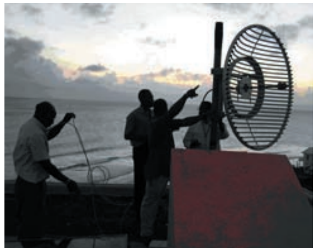
CBC personnel during installation of a repeater antenna.
